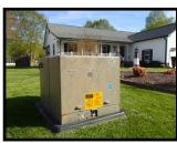
clude fences, shrubs, trees, storage sheds, and so on. Each pad has warning signs and guidelines for space needed around the transformer. Any obstruction can:
