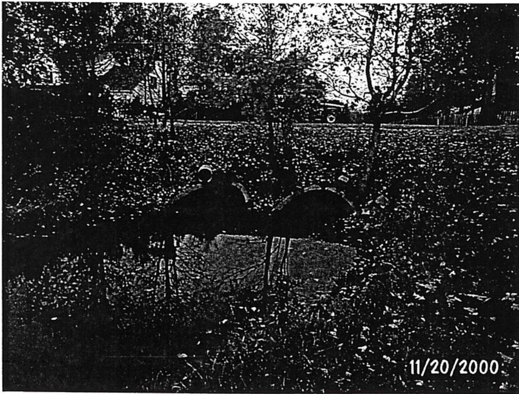
Photo #5 – View of twin elliptical pipes under Bridge Wood Drive looking north
