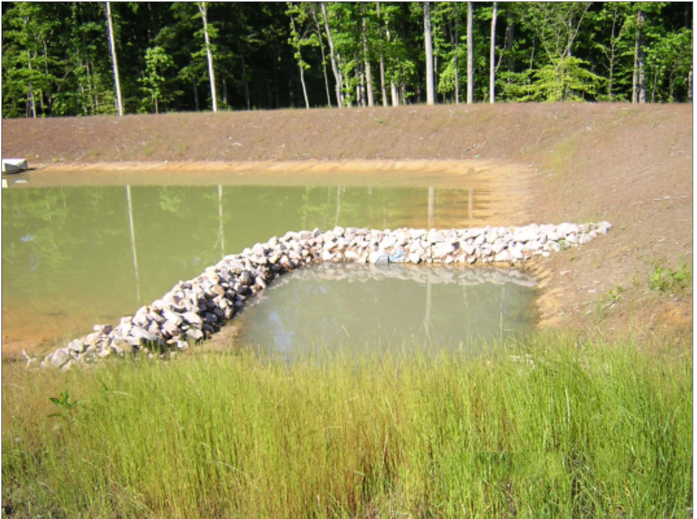
A traditional sediment forebay, such as the one above, encourages sediment to settle in one place, lowering maintenance costs. Below are drawings showing different ways the forebay can be configured.
