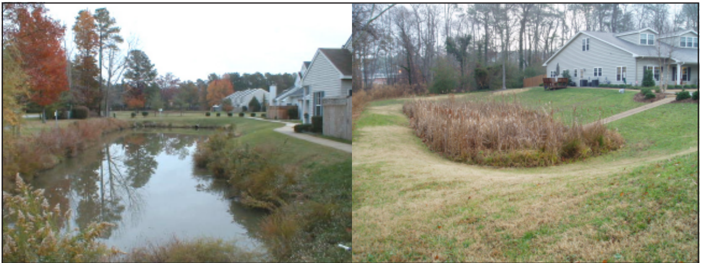
Simple depressions, ponds, or ditches that you see every day may actually be engineered facilities designed to improve water quality and reduce flooding.
