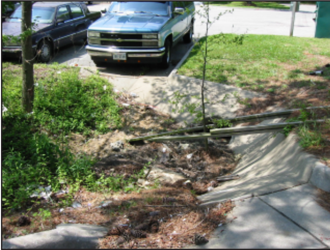
Not only are litter and debris unsightly, they can clog BMP components and create conditions perfect for insects.
