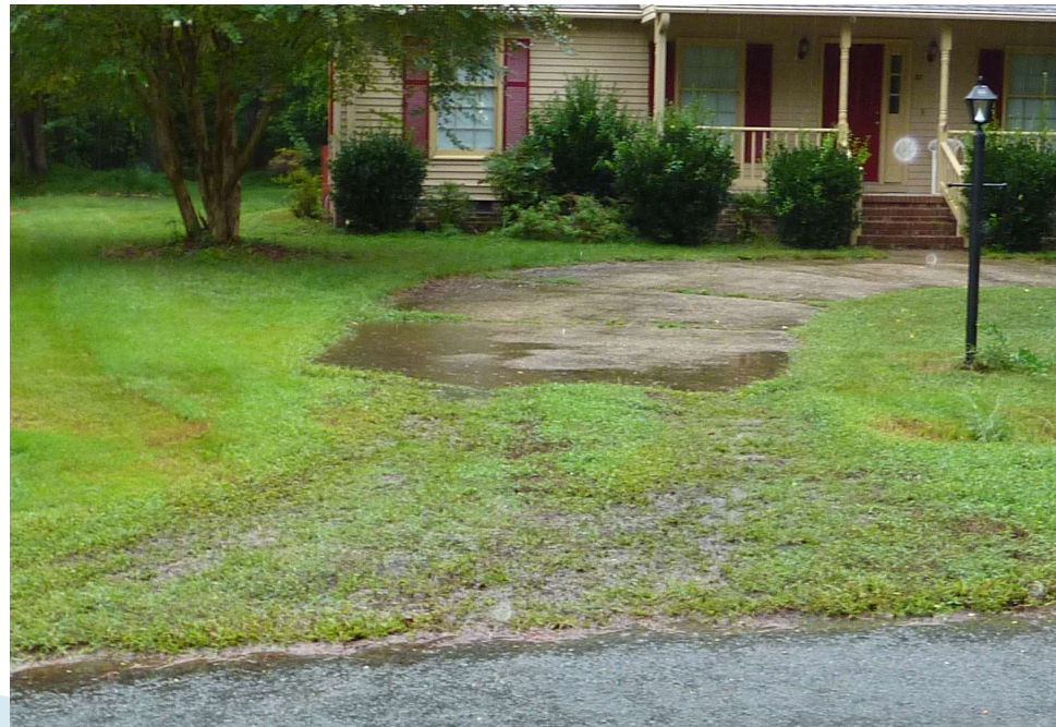
Overgrown Driveway Apron
